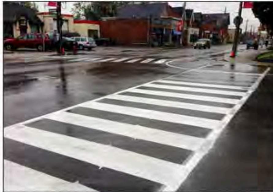
Crosswalk hatches and painted bumpouts at Locke and Herkimer (Image Credit: Jason Leach)
